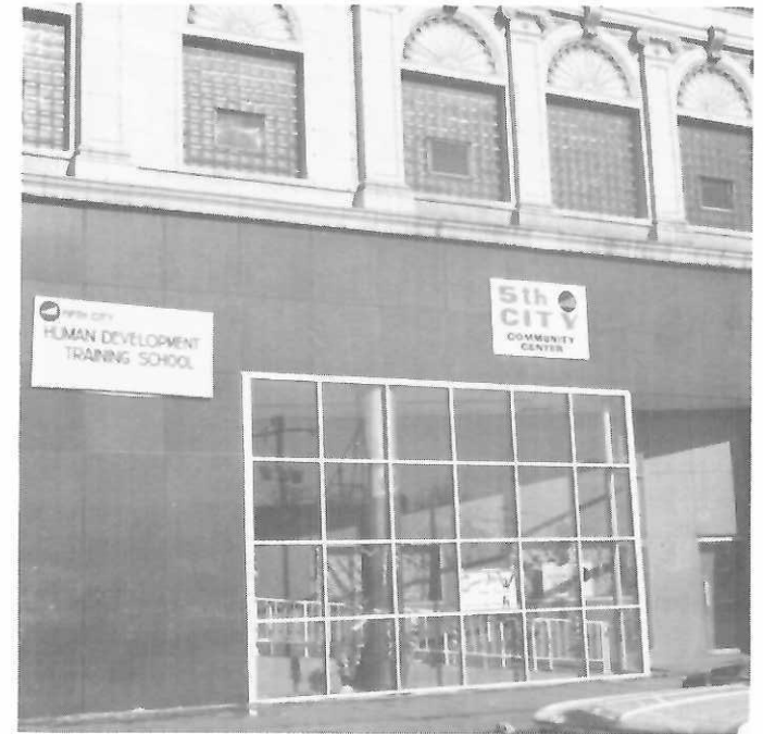
On the Iron Man Plaza, at 3300 West Jackson Boulevard, the Fifth City Community Center is now ready to rent for office or store space. Dances are often held in the Tom Washington and Allyn Adams Halls.
