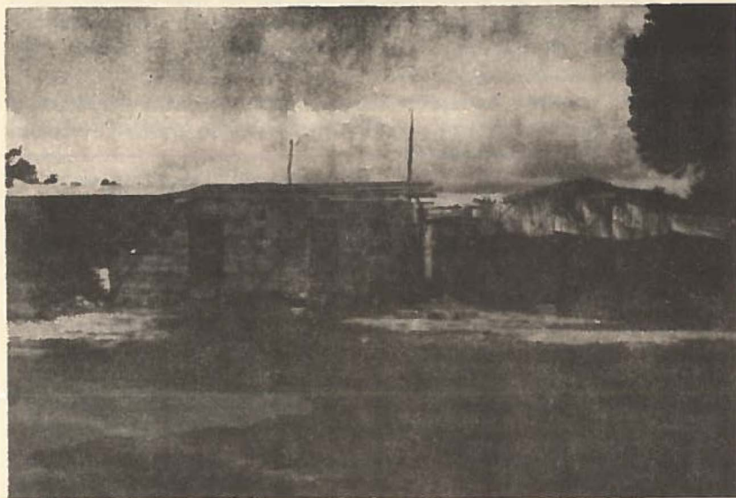
The old and the new — All the 34 villages in Muputi Location decided to build new nursery schools as one of their location wide projects.
