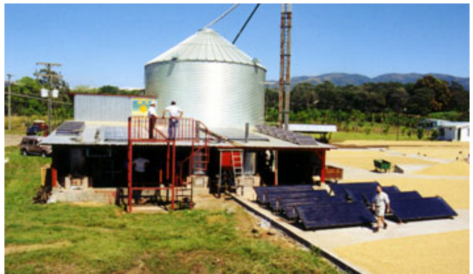
SOLAR-POWERED COFFEE DRYERS, MONTES DE ORO COOPERATIVE, COSTA RICA
