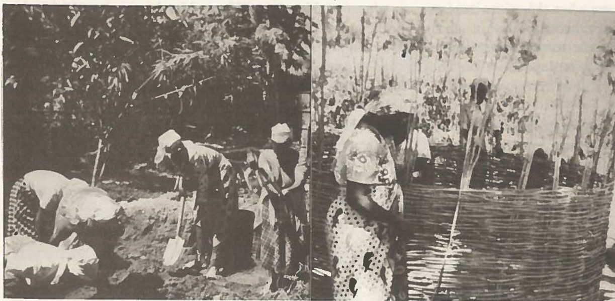
Digging the foundation and weaving the basket framework prepare for the water tank.
