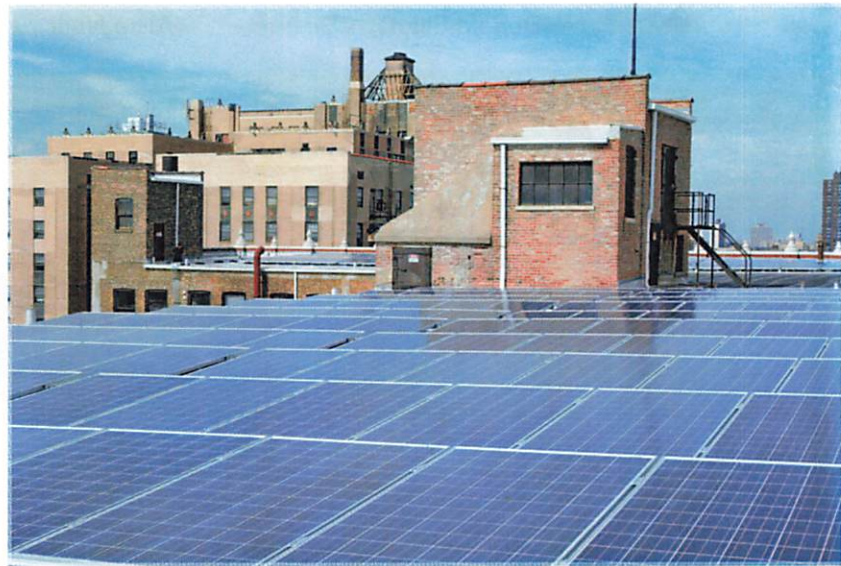
Rooftop shots before & after solar installation
