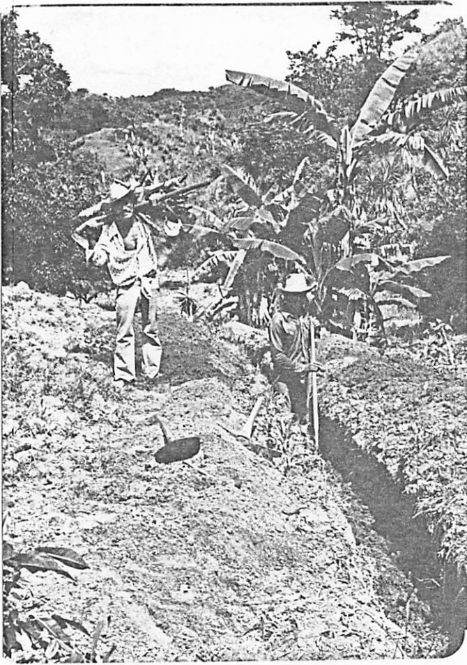
Digging the trenches for the irrigation pipeline - through the fields,
