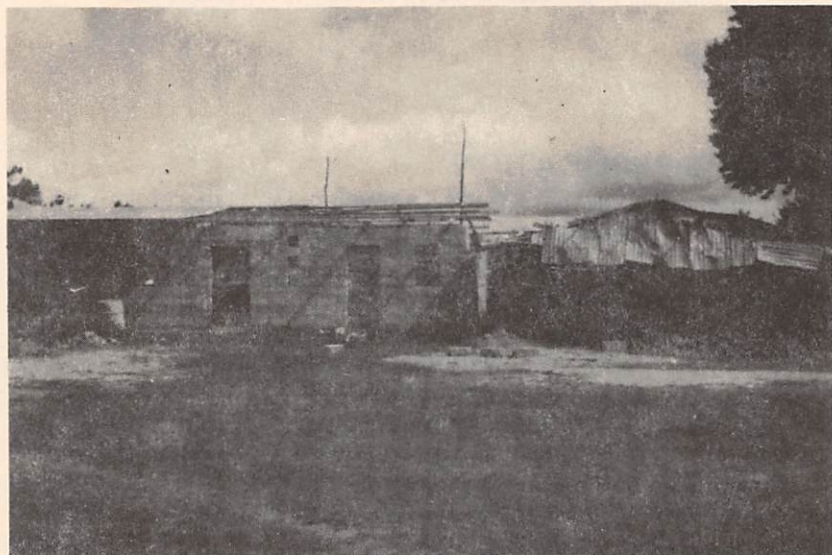
The old and the new — All the 34 villages in Muputi Location decided to build new nursery schools as one of their location wide projects.
