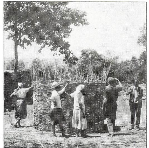
Water tank construction
