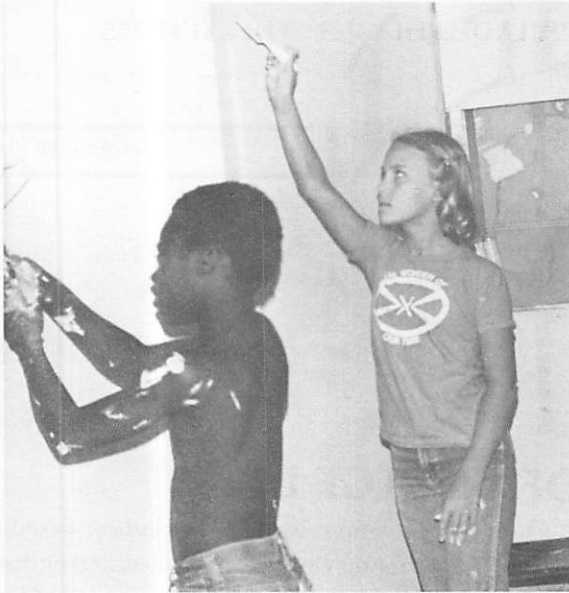
Emanuel Ward and Tina Slicker painting the walls (and other surfaces) as the students transform the Student House.
