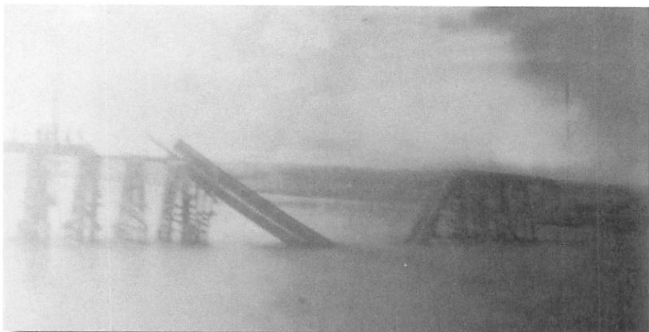
Canadian River Breaks Railroad Bridge 131
