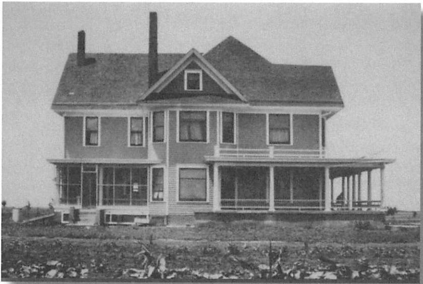
Hobart house during construction in 1913
