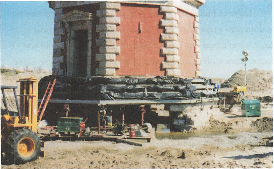
Moving the Hatteras Light House
