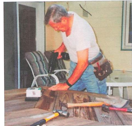
• Bob repairing a "found" hexagonal picnic table in Indianola
