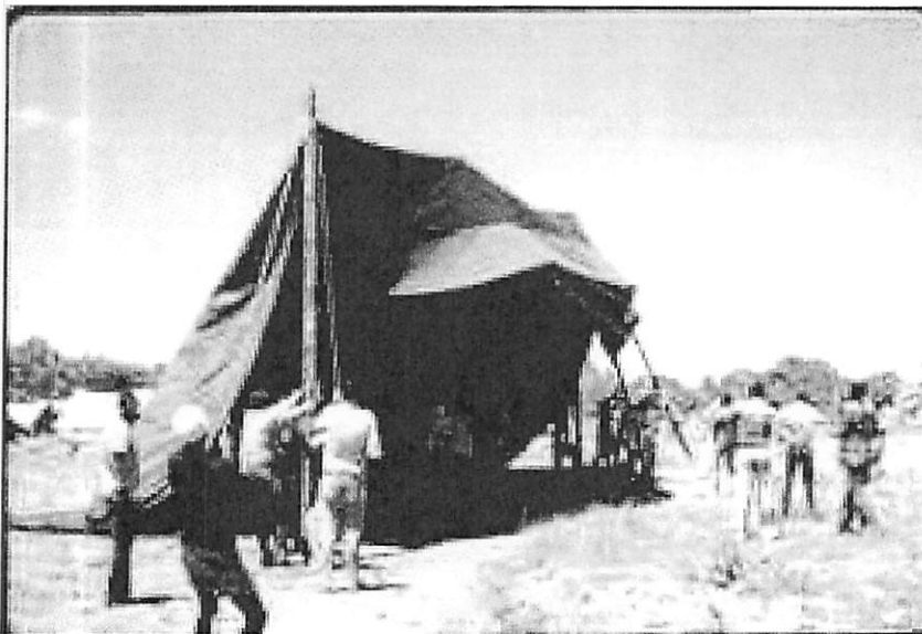
Figure 4. Building the assembly tent
