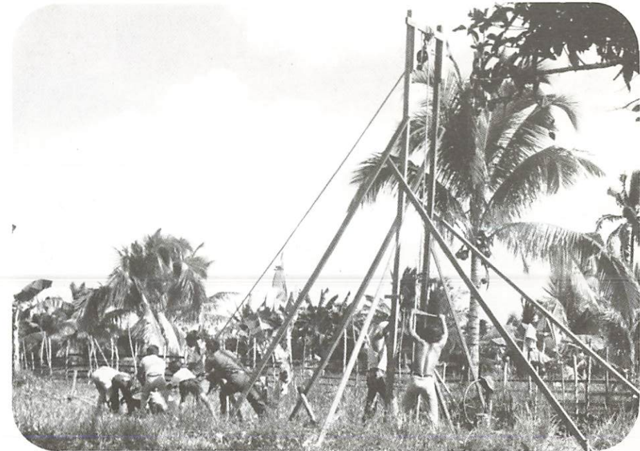
Drilling for water
