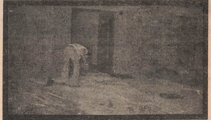
Workmen finishing up the Gymnasium floor for the KNIGHTS' basketball season.
