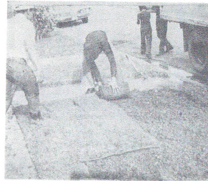
Rolling Out New Sod
