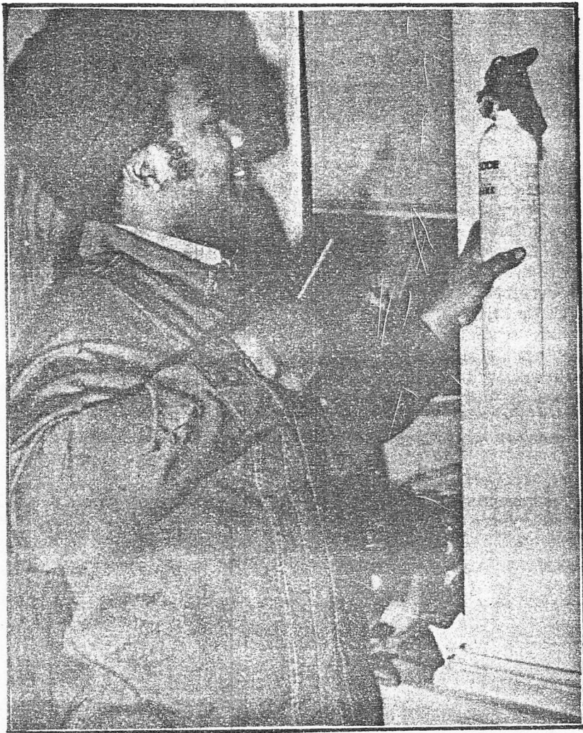
Jaycee Installs Fire Extinguisher
