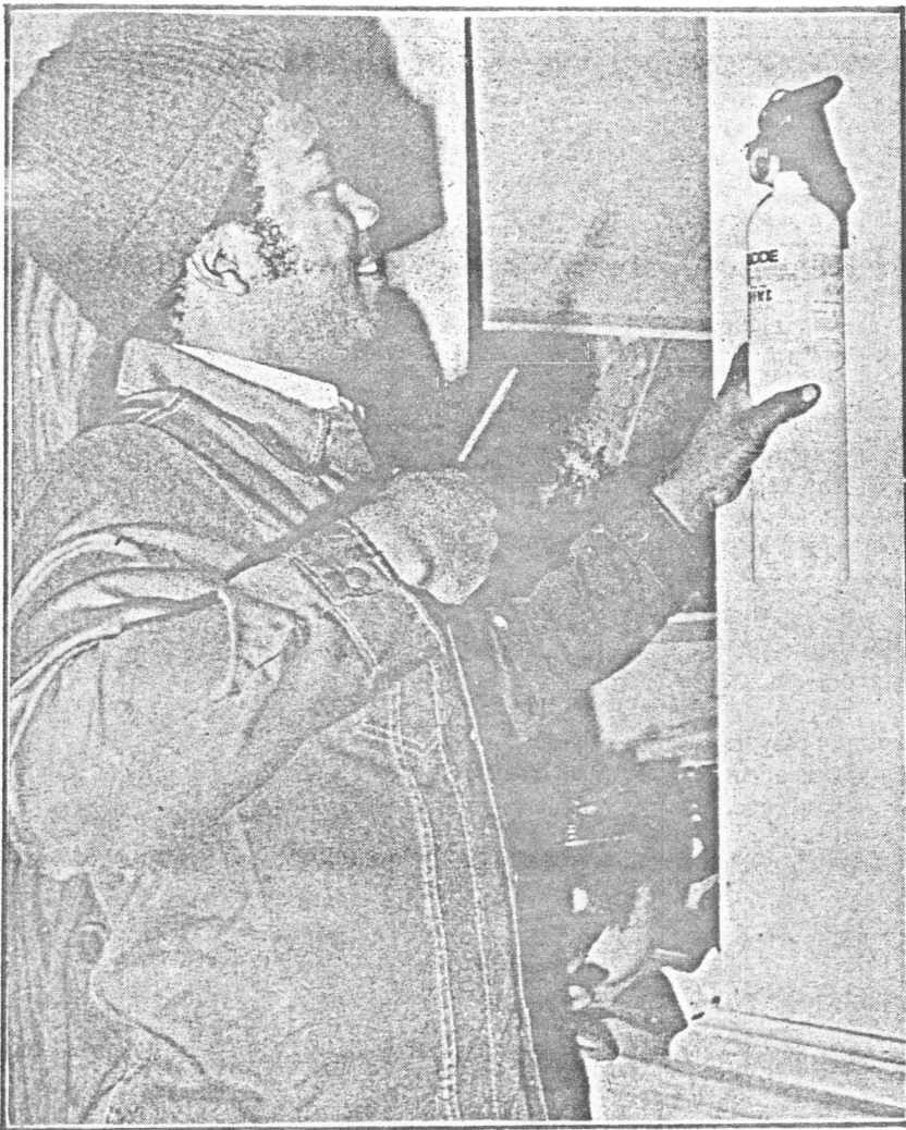
Jaycee Installs Fire Extinguisher
