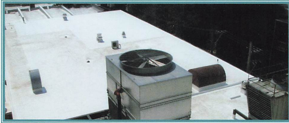
Before and after photos of the roof at 4750 N. Sheridan Road.
