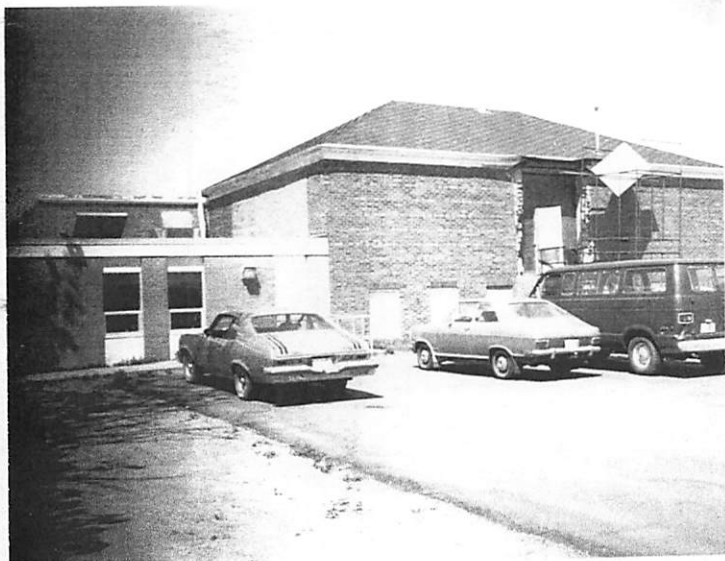
GRADE SCHOOL WITH NEW ROOF
