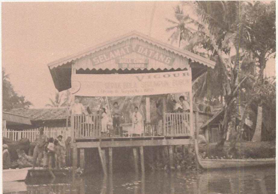
The rebuilt boat landing in Bubun welcomes residents and visitors
