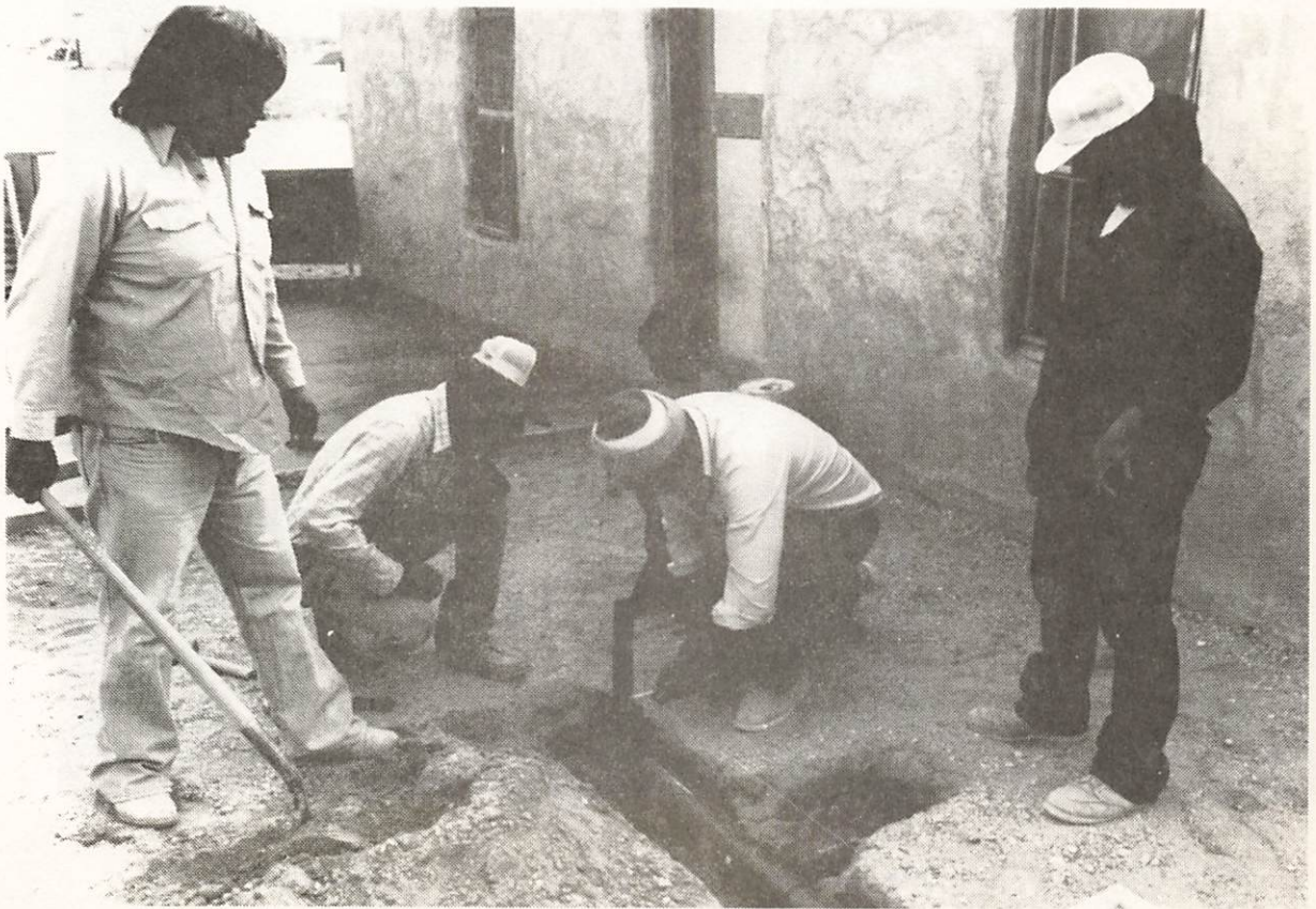
PISINEMO ADOBE CREW STARTING ANOTHER HOME REHAB PROJECT.
