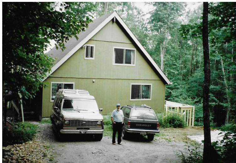
Rear view of Wolfe Laurel Home with downstairs bedroom under construction
