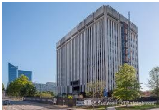
Albermarle Building Mental Health Division was on the 11 th Floor
