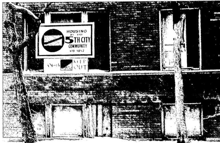
5th City building ready for rehabilitation.
