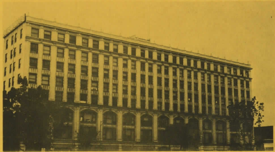
Kemper Building, Chicago, Illinois
